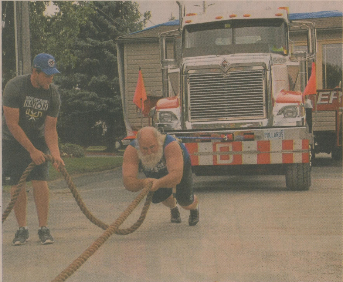
Strongman Kevin Fast hauls a small house 30 metres on the last leg of its trek to a new location in Brighton, Ont. The two-bedroom cottage was donated to Habitat for Humanity. His son, Matthew, handles the rope to guide him.
